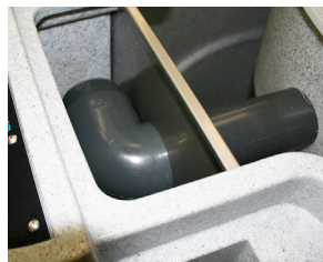
Figure 17.3 - By-pass in operation
